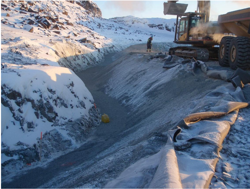
Photos 3: Photo of the Doris North Diversion Berm; excavator placing crush along the crest. Bentonite chips along the base of the key-trench extend up to the jerry-can.
