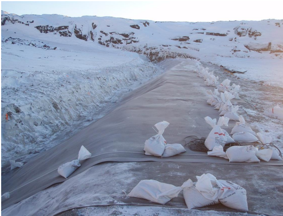
Photos 4: Extent of current HDPE placement; approximately 100m of placement to date.
