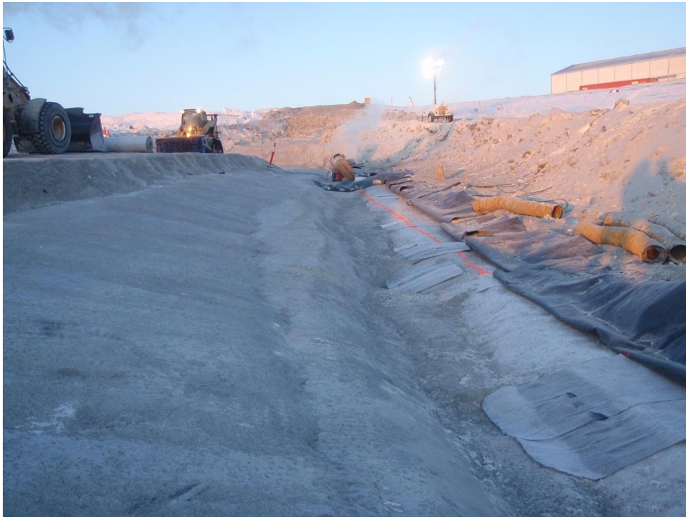
Photo 6: Dental cleaning from chainage 1+50 to 1+90 at the dam. Patches were cut and placed over tears; no bentonite has been applied at this point.
